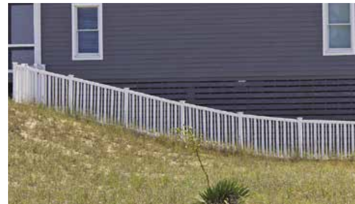
Example of Rackability (follows incline)
